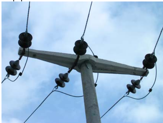
Fig. 9. Top of angle-straining pillar ( 10 kV overhead line, “ KRAVLJI DO - ŠLJIVOVAC” )
